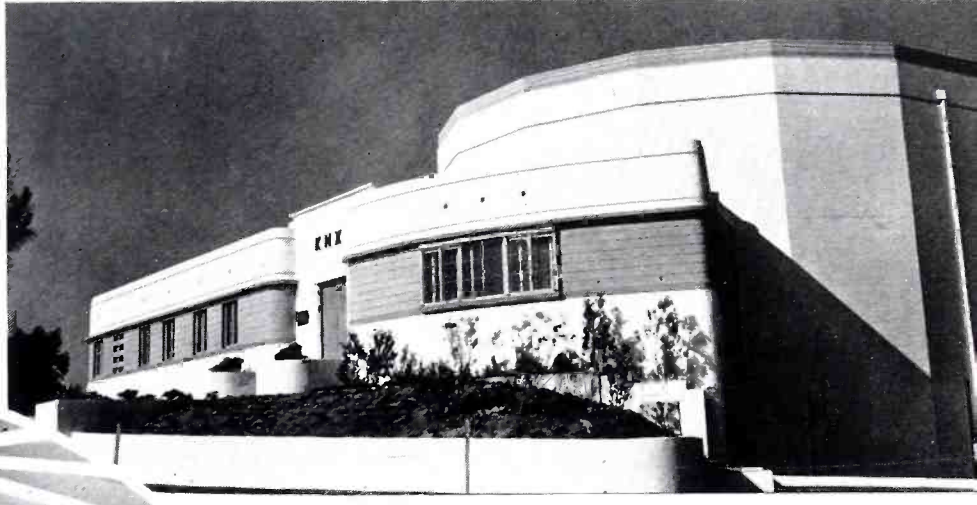
▲ Modernistic KNX Transmitter House.
